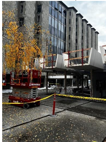
Plaza Abatement Complete
