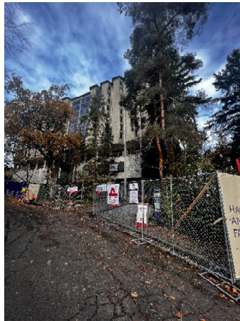
South Entrance Scrim Install
