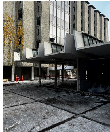
Podium Skylight Removal
