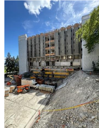
South Tower Rooftop Demo
