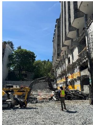
Casework Removal North Tower
