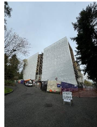
South Tower Scaffold
