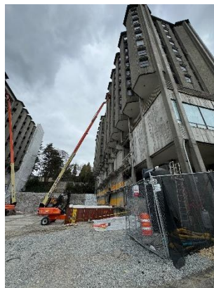
North Tower Abatement
