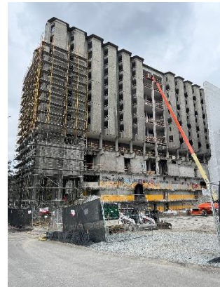
South Tower Abatement
