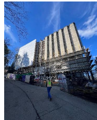
South Tower Scaffold
