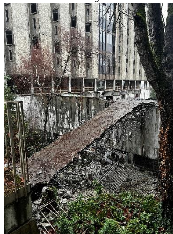
Podium Bridge Demolition
