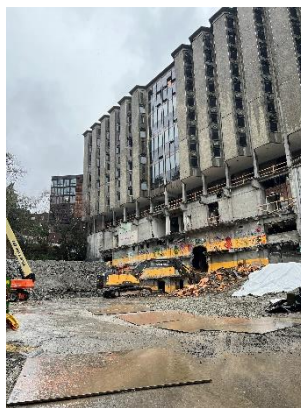
Podium Debris Removal
