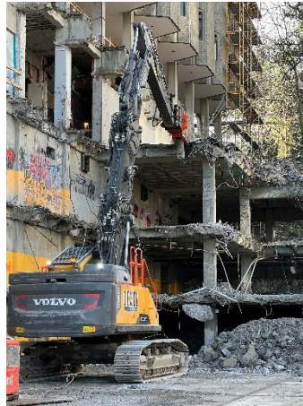
West Podium Demolition
