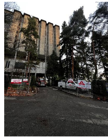
Debris Load out From Podium
