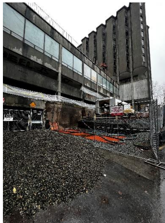
Rock Delivery East Entrance
