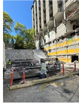
South Tower Panel Removal
