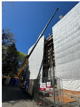
South Tower Panel Abatement
