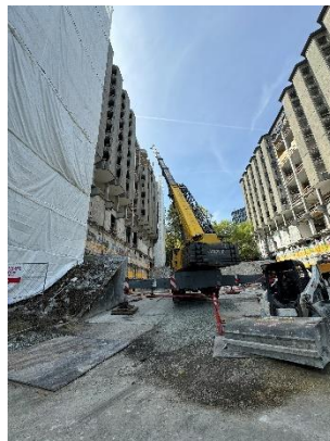
South Tower Panel Removal
