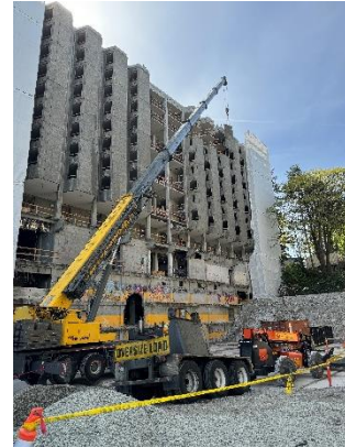
South Tower Panel Removal
