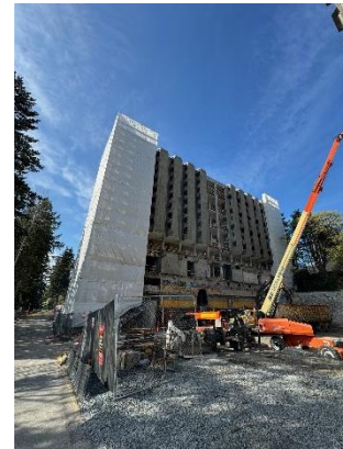
South Tower Scaffold
